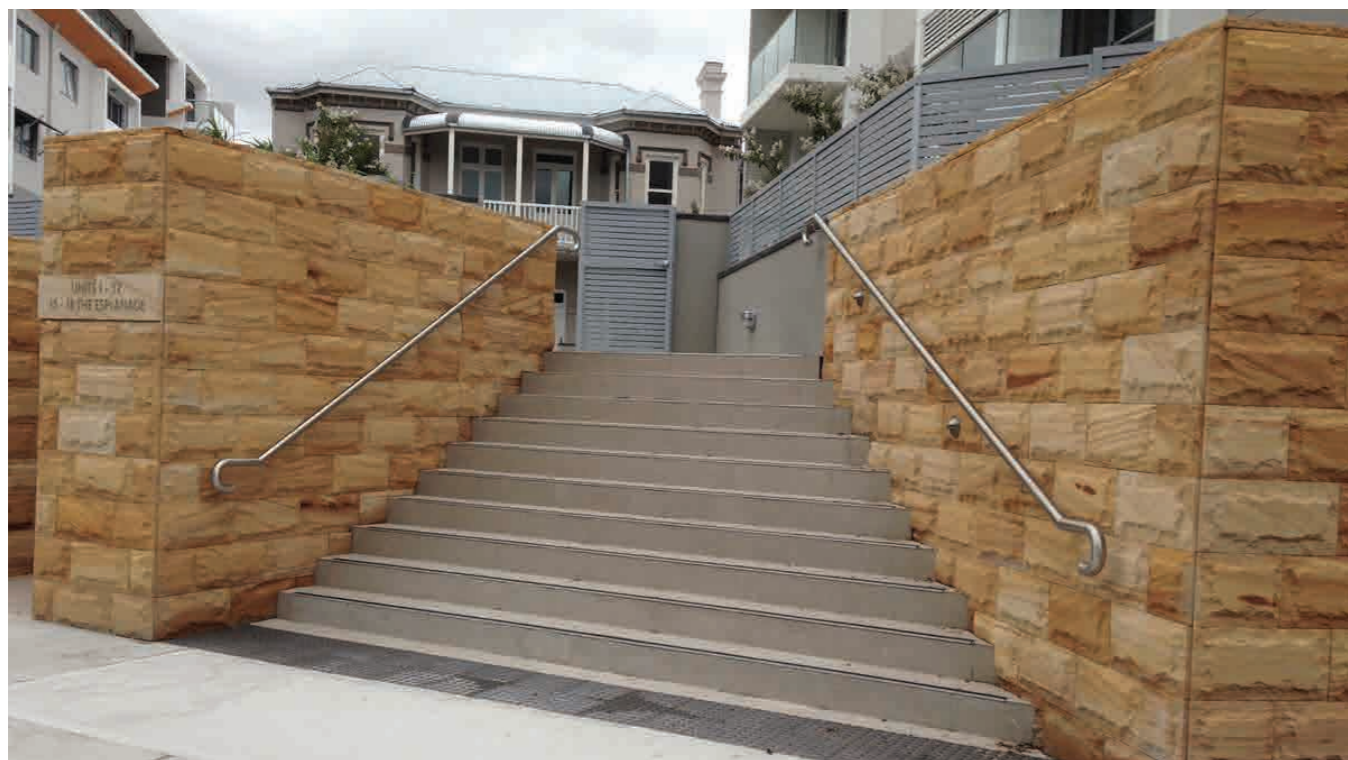
SANDBLASTED CHIPPED EDGES
